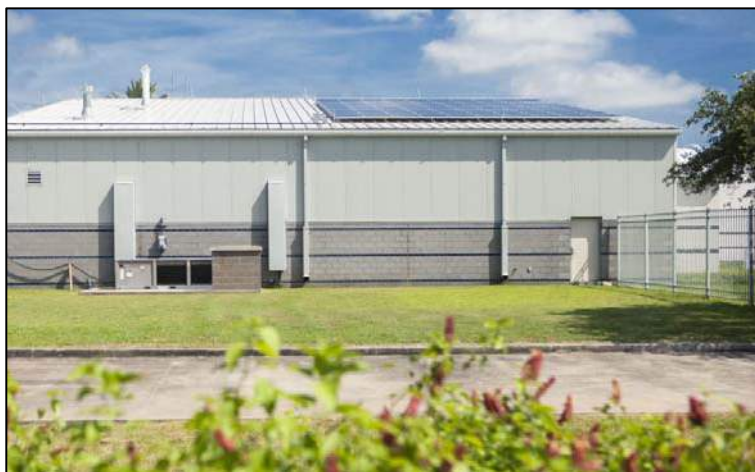
South elevation of the Sea Center Texas office and exhibit building showing solar panels on roof.
