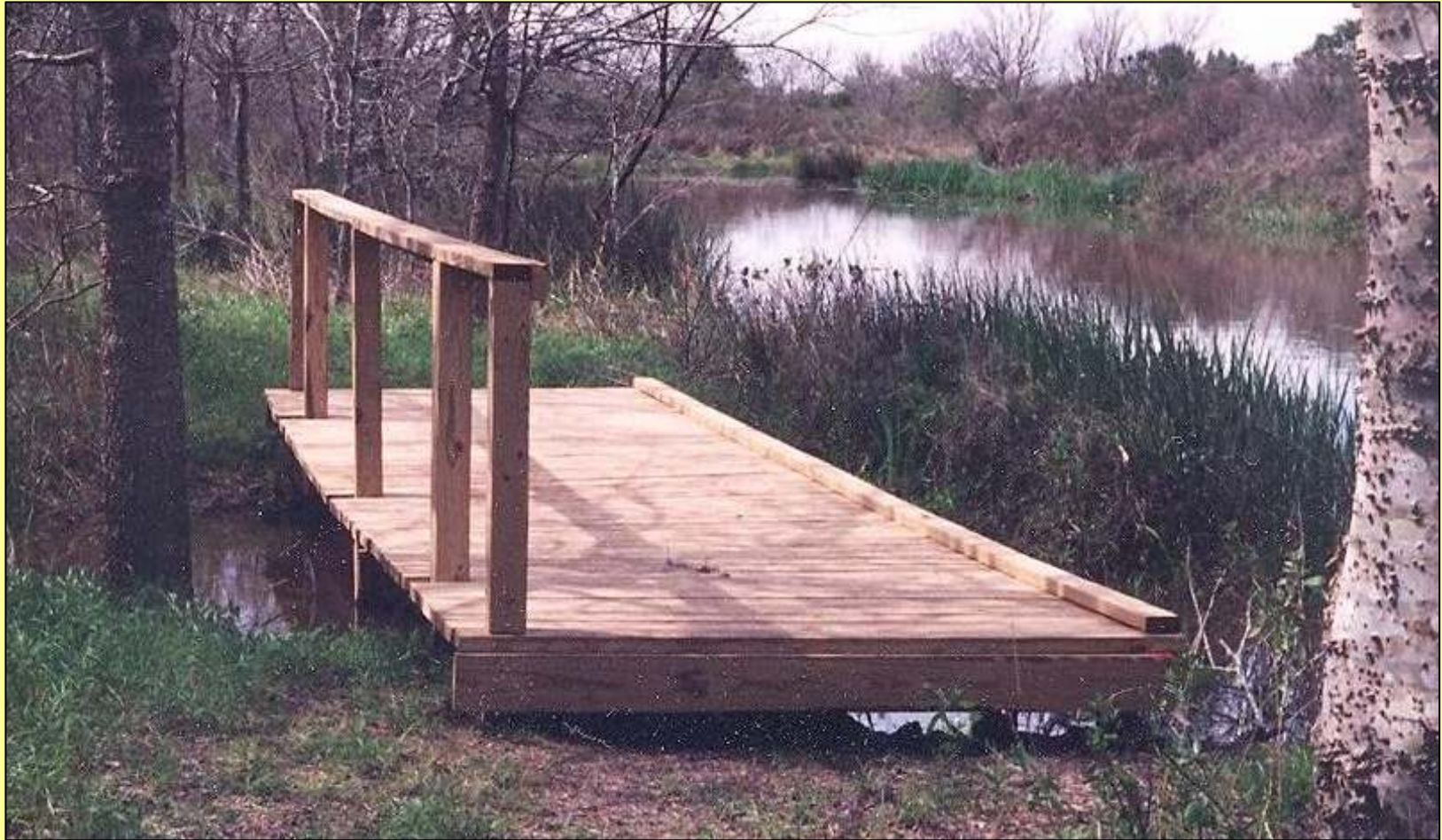
First bridge on Bobcat Woods Trail
