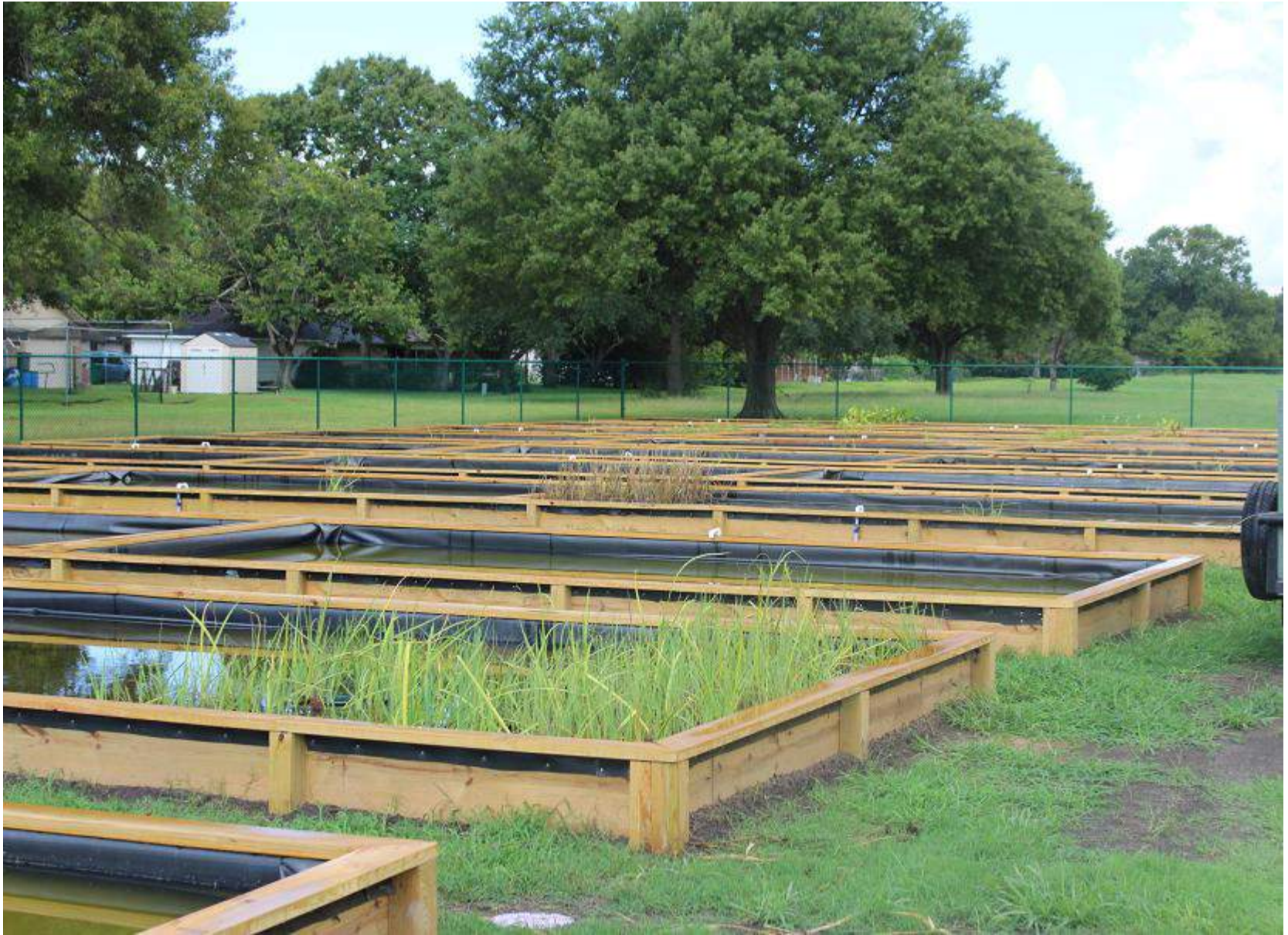
Above-ground plastic-lined ponds used for growing out potted wetland plants.
