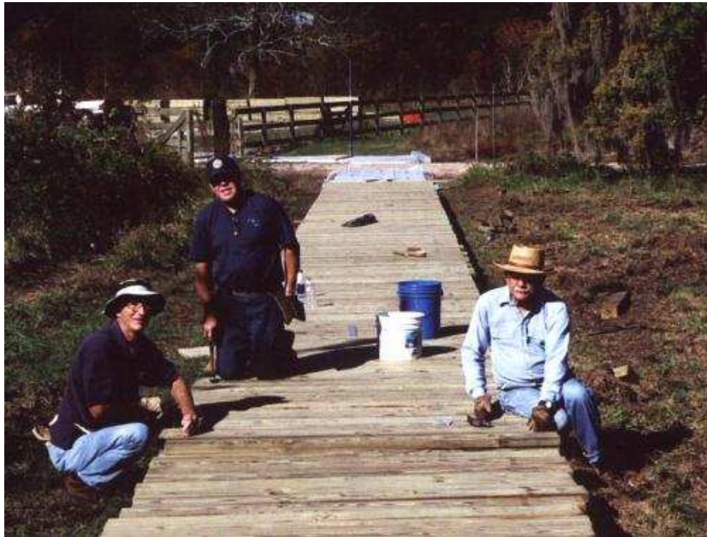
Boardwalk Construction. Photo by Jerry Krampota, 2004.
