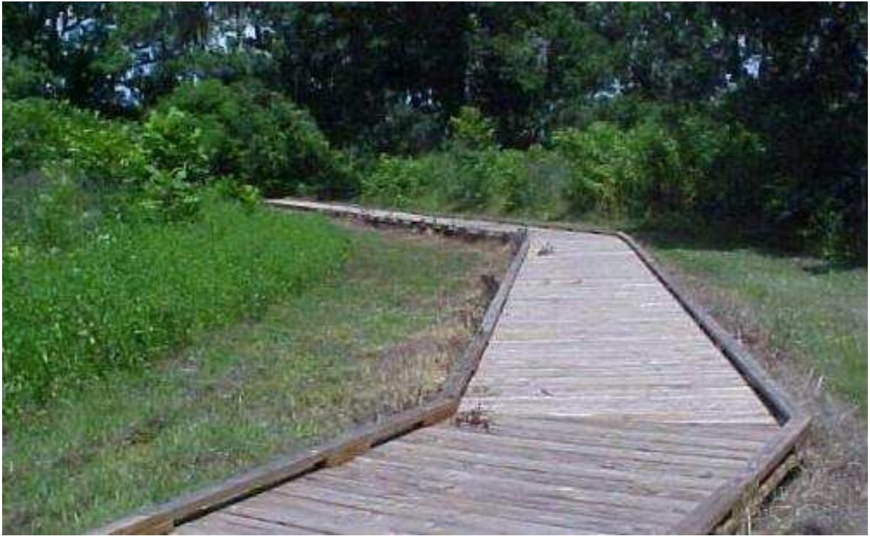
The finished boardwalk, June 2005
