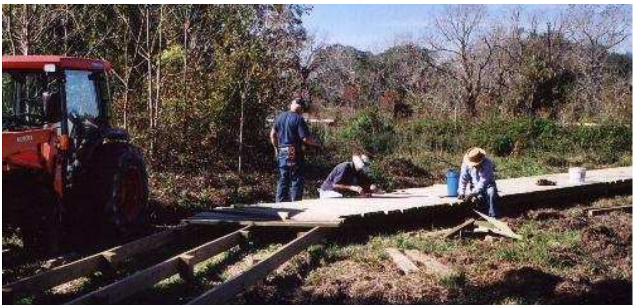
Boardwalk Construction. Photo by Jerry Krampota, 2004.
