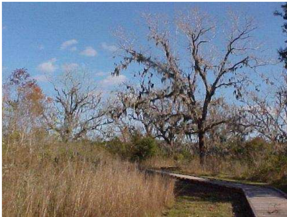
The finished boardwalk, June 2005
